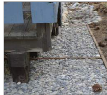
Gravel area under a gutterless roof
