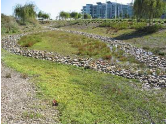
Extended detention ponds are basins whose outlets have been designed to detain the stormwater runoff from a water quality design storm for some minimum time (e.g., 48 hours) to allow particles and associated pollutants to settle.
