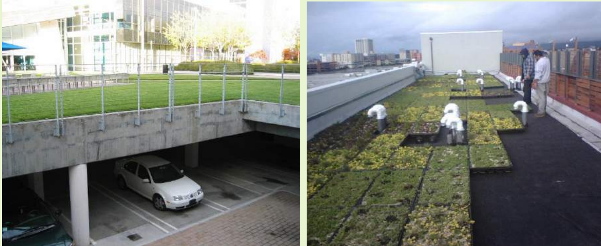
Figure 6-44: Parking Lot with Turf-Covered Intensive Green Roof, Google building, Mountain View; and Modular Extensive Green Roof installation, Emeryville. (Credit: EOA, Inc.)
