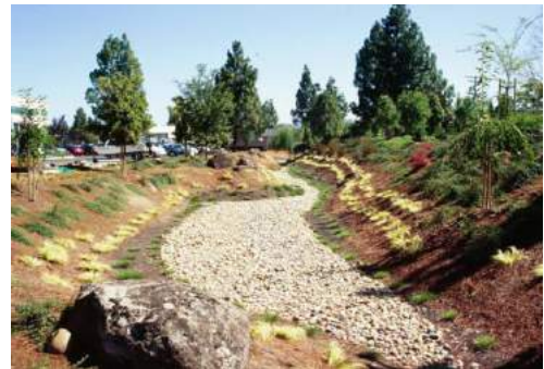
Figure 8-7: Extended Detention Basin, Palo Alto
