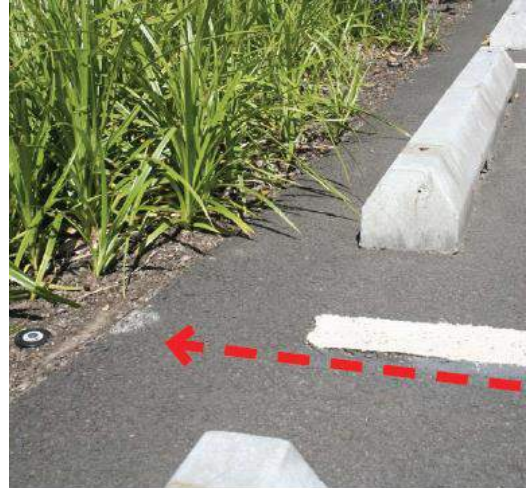
Figure 5-16: Stormwater runoff enters the stormwater facility through the 3-foot space between these wheelstops. The design could be improved by providing more drop in grade between the asphalt and landscape area. (Credit: SMCWPPP, 2009)
