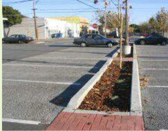
Figure 6-34: The City of Menlo Park used pervious concrete for parking stalls and standard paving in the drive aisles in this public parking lot. (Credit: City of Menlo Park)
