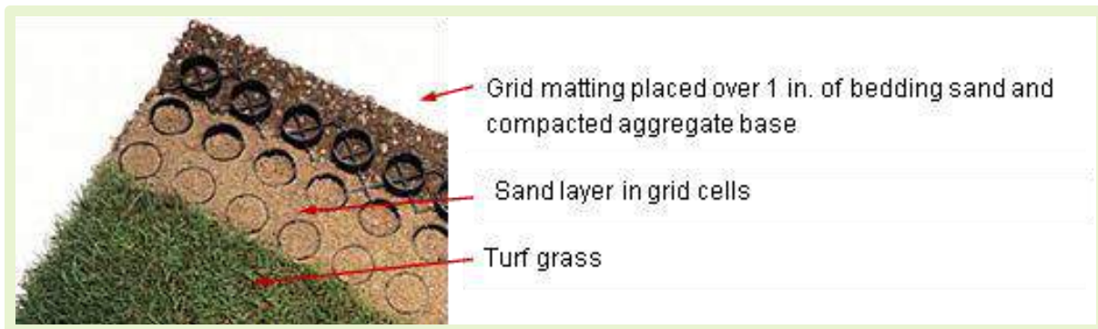
Figure 6-43: Plastic Reinforced Grid Paving for Occasional Vehicular Use or for Emergency Access Lanes (Credit: Santa Clara Valley Urban Runoff Pollution Prevention Program). Note: Sand and turf grass can be replaced with ASTM No. 8 aggregate in cell openings.
