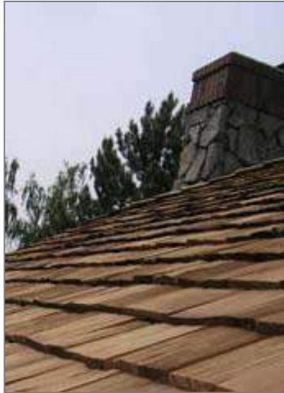
Wood shingle roof Courtesy of Gutter Glove
