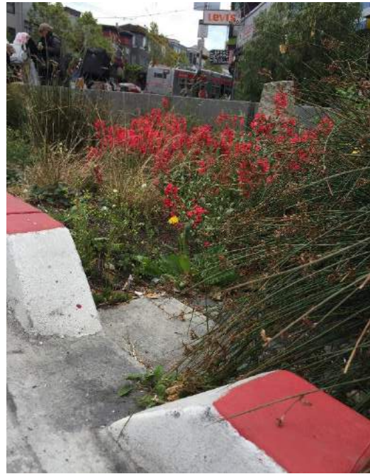
Figure 5-11: This standard curb cut in San Francisco has angled sides, a depressed throat and a 2-inch drop off to a splash apron. (Credit: EOA, Inc.)
