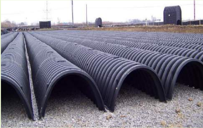
Figure 6-52: Photo of subsurface retention/infiltration system installation under a parking lot (Credit: CONTECH Engineered Solutions)
