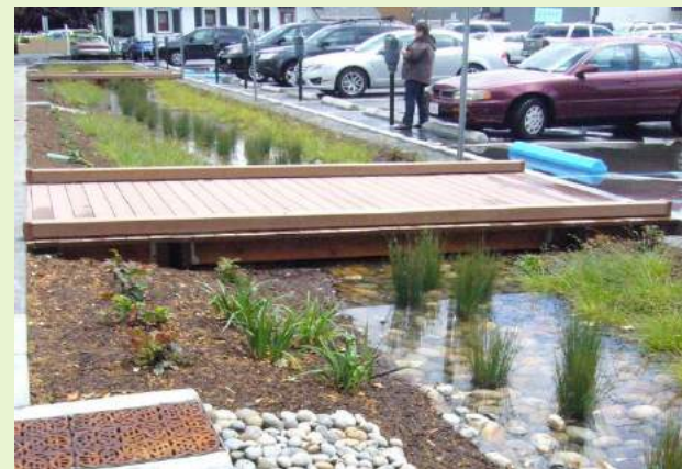
Figure 6-3: Bioretention area in a multi-family residential property in Redwood City (top; Credit: EOA, Inc.) and in a parking lot in Burlingame (bottom; Credit: SMCWPPP)
