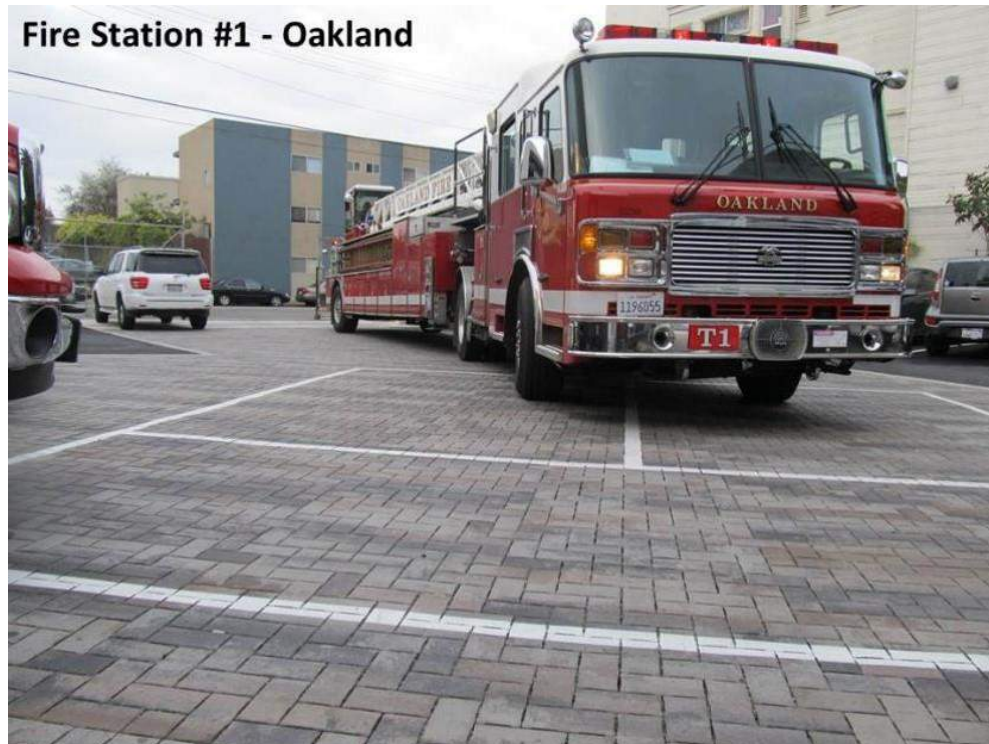
Figure 4-9: Installation of permeable interlocking concrete pavers in Oakland. Water infiltrates through gravel in the joints between the pavers. (Courtesy of the City of Oakland)
