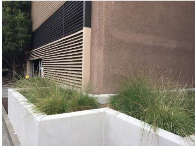
Figure 8-4: Flow through planter in Emeryville (Credit: EOA, Inc.)
