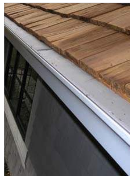
This gutter is covered by a fine mesh gutter guard to keep debris out. Courtesy of Gutter Glove
