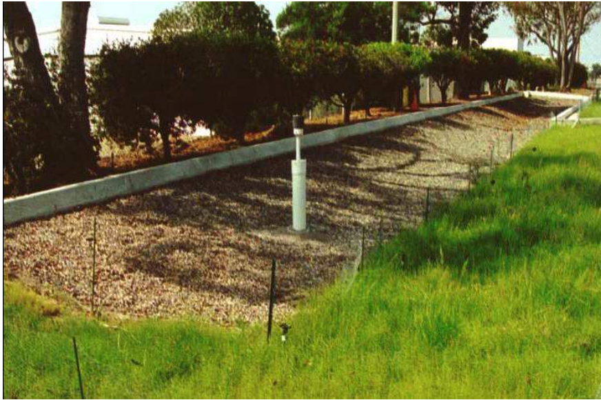
Figure 8-6: Infiltration Trench (Credit: CASQA)
