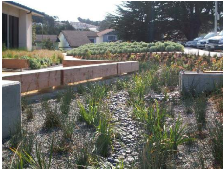
Figure 8-3: Bioretention Area in Daly City (Credit: SMCWPPP)
