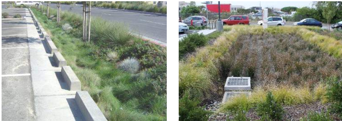
Figure B-2: Examples of Bioretention Areas
