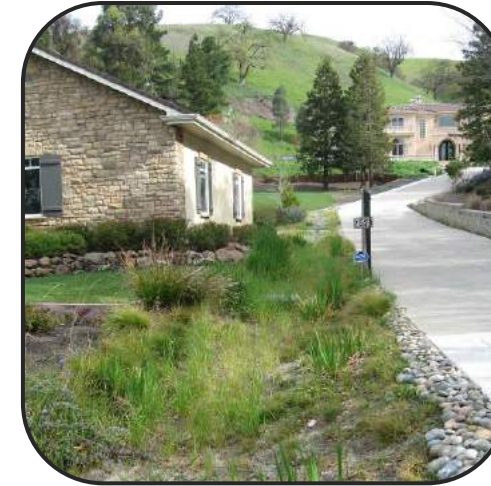
Large Residential Rain Garden
