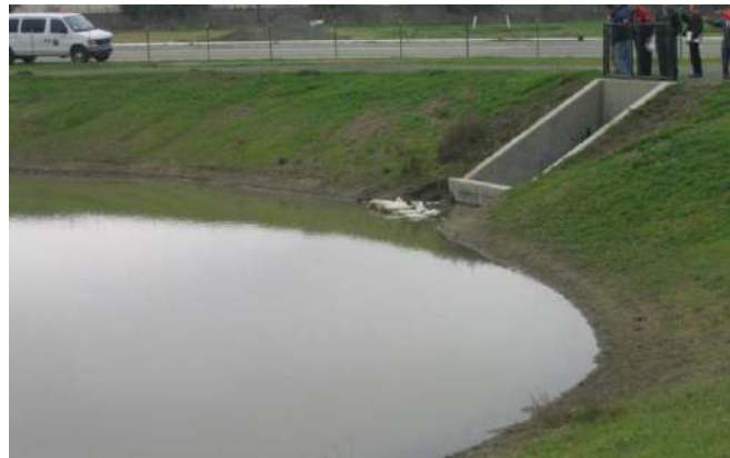
Figure 5-6: Detention pond used for hydromodification management.
