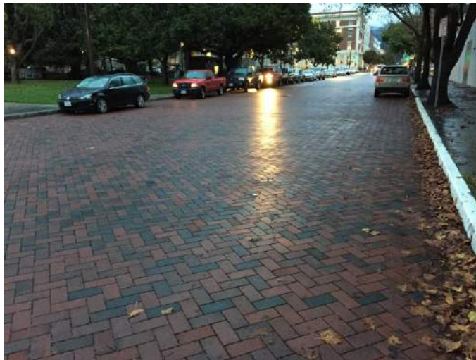
Figure 8-8: Permeable pavers in Berkeley (Credit: EOA Inc.)
