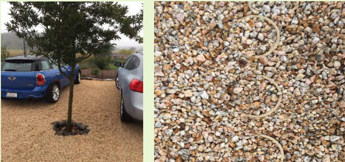
Figure 6-41. Reinforced grid paving in an overflow parking lot in Napa. (Credit: EOA, Inc.)
