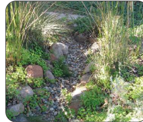
Dry creek infiltrates and conveys runoff.
