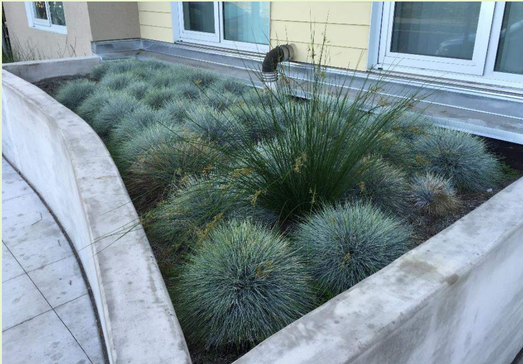
Figure 6-12: Flow-through planter (Credit: EOA, Inc.)
