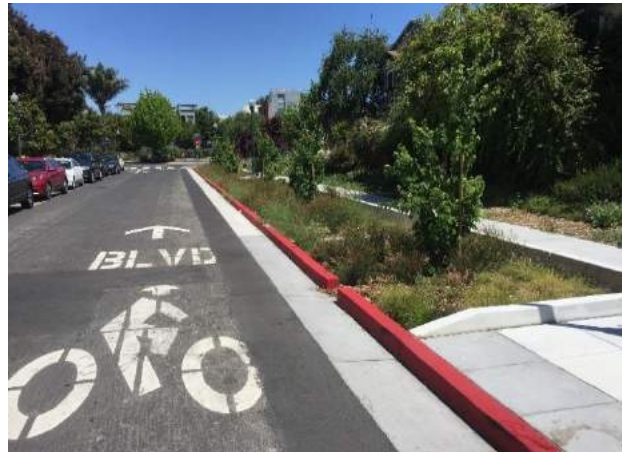
Figure 9-2: After: Parking moved to the west side of the street and the landscape strip widened into a Bay-Friendly bioretention area with new trees.
