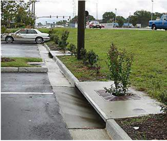
Proprietary Tree Well Filters typically consist of a pre-cast concrete box with a small tree or shrub planted in engineered media with surface mulch.
