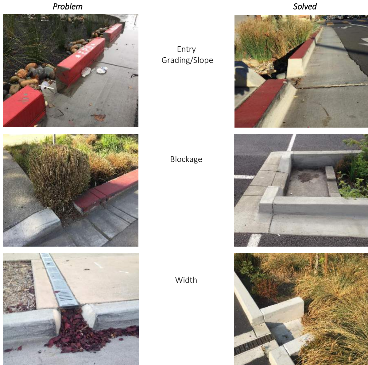
Figure 5-8 – Examples of common design problems with inlets of treatment measures. (Credit: EOA, Inc. and City of Mountain View)
