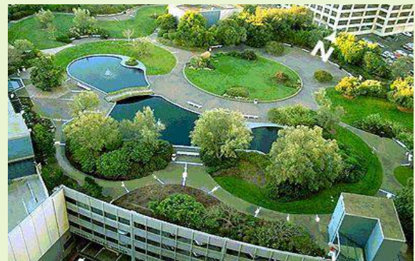
Figure 6-45: Top: Extensive Green Roof at YouTube Headquarters, San Bruno (Courtesy of William McDonough & Partners); Bottom: Intensive Green Roof, Kaiser Center Parking Garage, Oakland. (Credit: Gene Anderson)
