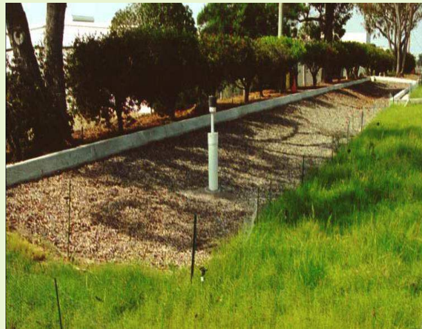
Figure 6-27. Infiltration Trench (Source: CASQA, 2003)
