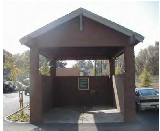
Central Wash Area in Apartment Complex Parking Lot. Source: City of Palo Alto, California
