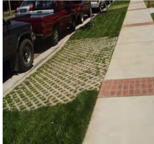
Use of reinforced grass pavement (“grasscrete”) allows for pedestrian access without vegetation damage and reduces runoff through infiltration. Photo: Alameda Countywide Clean Water Program
