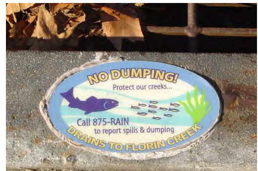
Pre-fabricated inlet marker Photo source: County of Sacramento
