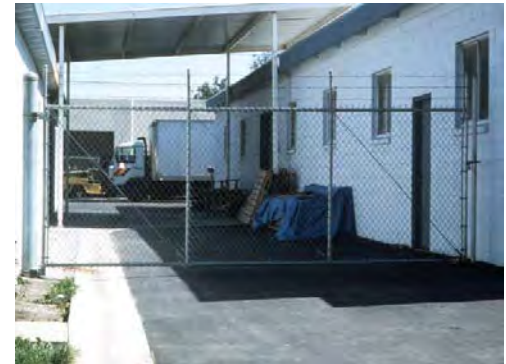
Paved and covered outdoor work area. Photo: CASQA, 2003
