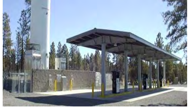
Covered fueling area. Photo source unknown
