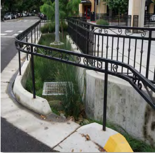
Figure A: Urban Infiltration Trench BMP
