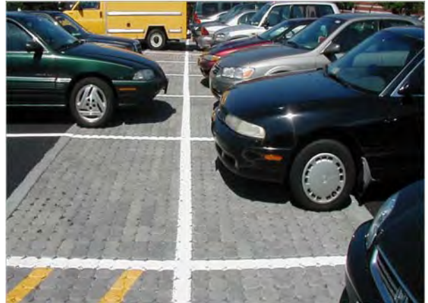
Pavers in parking lot. Photo: City of Emeryville
