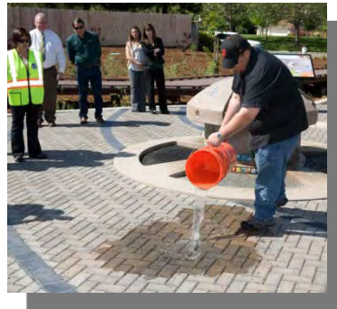
Porous Pavement at Elk Grove-Rain Garden Plaza
