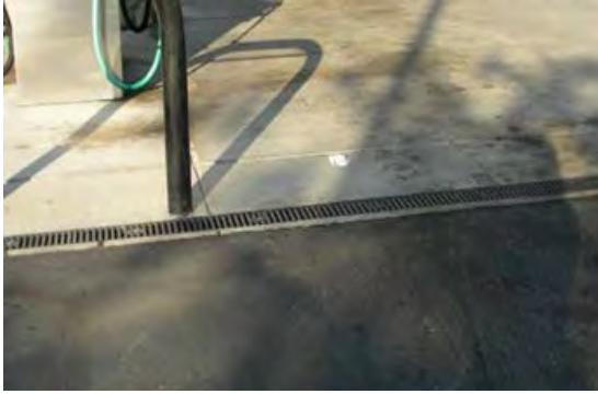
Interceptor drains on the fueling pad perimeter at this retail gasoline outlet in Folsom catch spills and incidental contaminated wash water and direct it to an onsite 750-gal underground containment tank.
