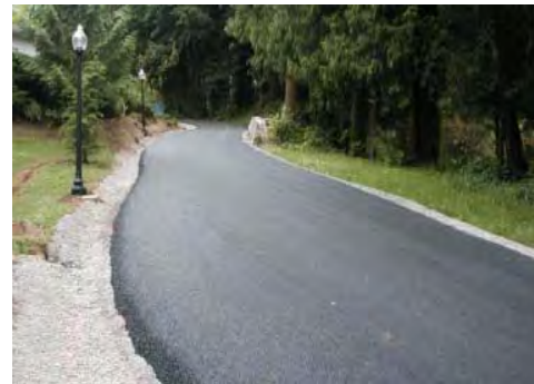
Pervious asphalt roadway. Photo: City of Portland
