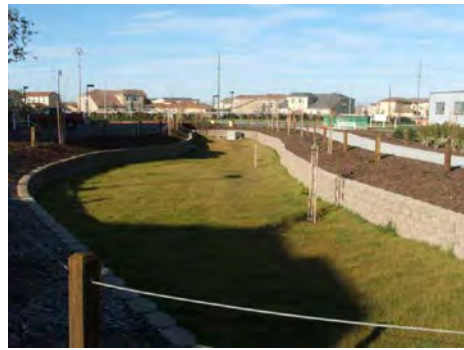
Photo: Bilby Road, The City of Elk Grove
