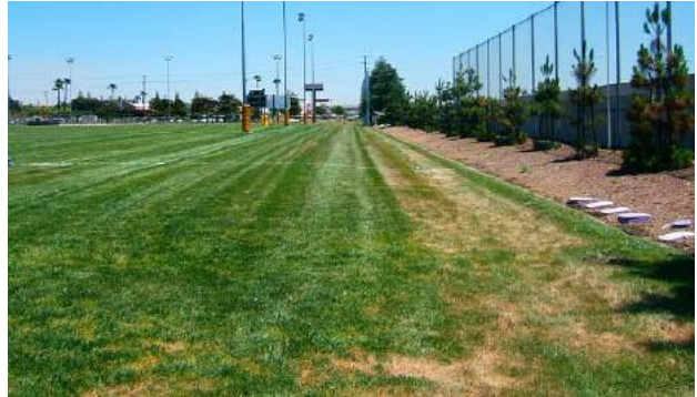
Photo 3-3. This sports field in Dublin also functions as a stormwater detention area.
