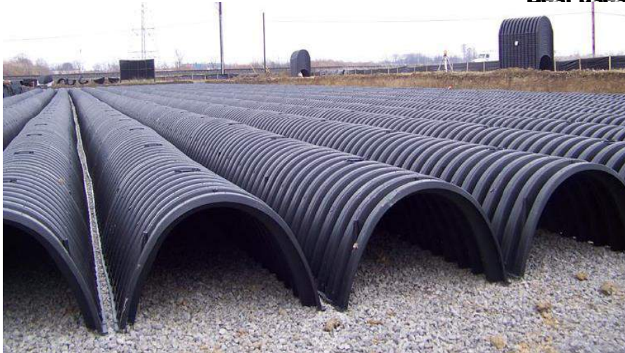
Photo 6.11-1. Subsurface retention/infiltration system installation under a parking lot.
