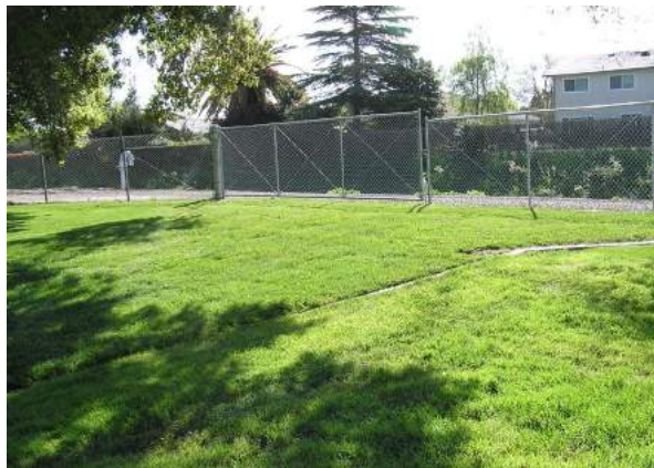
Photo 3-2. Pleasanton Sports Park includes this turf block fire access road.
