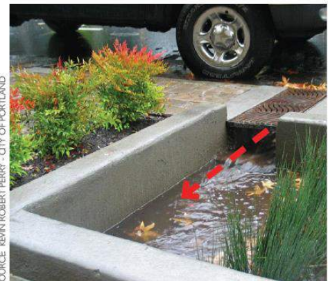
Photo 5-7. A grated curb cut allows stormwater to pass under a pedestrian egress zone to the stormwater facility.
