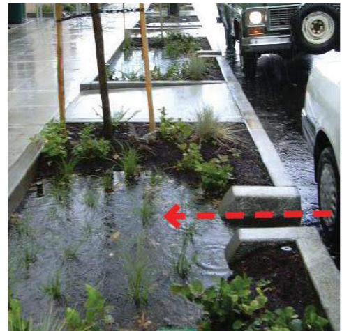
Photo 5-5. The side wings of this standard curb cut help retain the side slope grade on each side of the curb cut opening.
