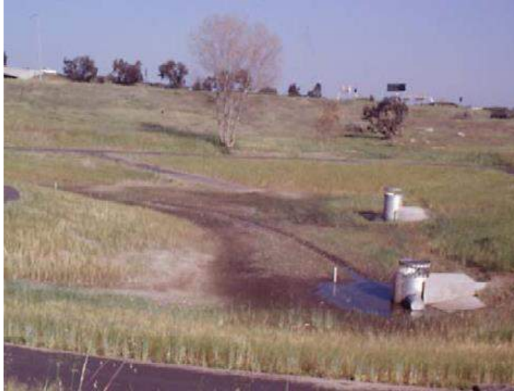
Photo 6.5-1. Extended detention basin.
