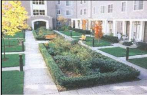
Typical Bioretention Area
