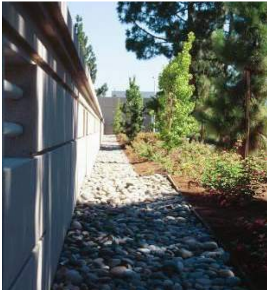
Photo 6.4-2. Infiltration trench next to parking structure, Palo Alto.
