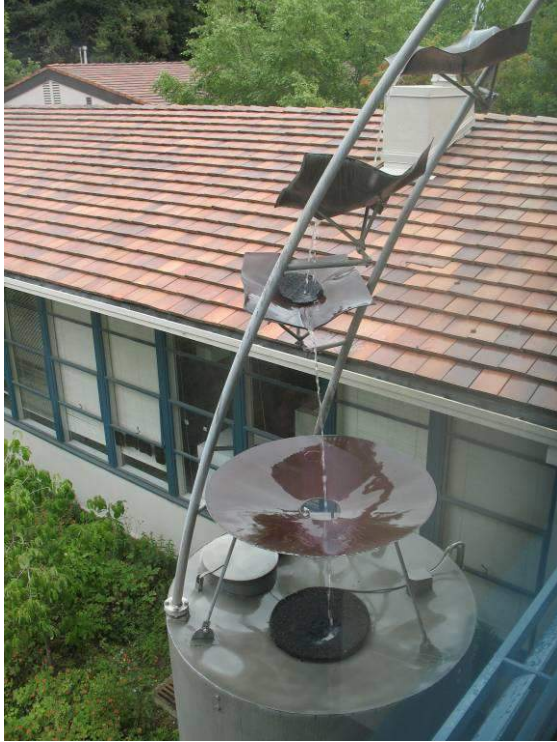
Photo 6.8-1. Rainwater is collected and used for flushing toilets at Mills College, Oakland.
