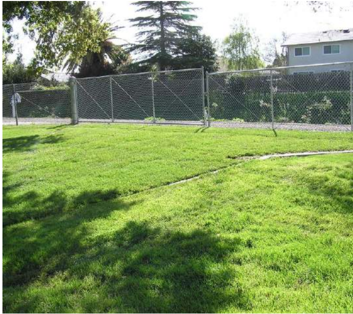
Photo 6.7-1. Turf block fire access
