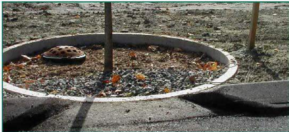
Photo 6.3-2. Non-proprietary Tree Filter with Overflow Bypass. Source: University of New Hampshire Environmental Research Group, 2006
