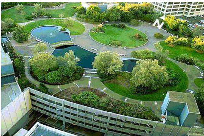
Photo 6.8-4. : Intensive Green Roof at Kaiser Center, Oakland
