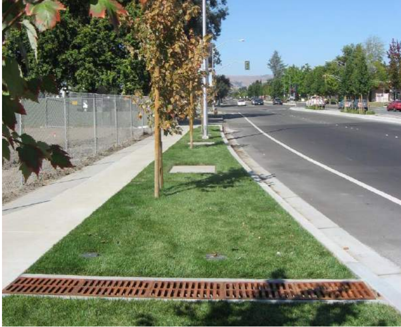
Photo 6.3-1. Non-proprietary tree well filters in Fremont use bio-retention soils with an infiltration rate of 5 to 10 inches per hour. Spacing the units closely together provides a total tree well filter surface area that is 4 percent of the impervious surface area from which stormwater runoff is treated.
