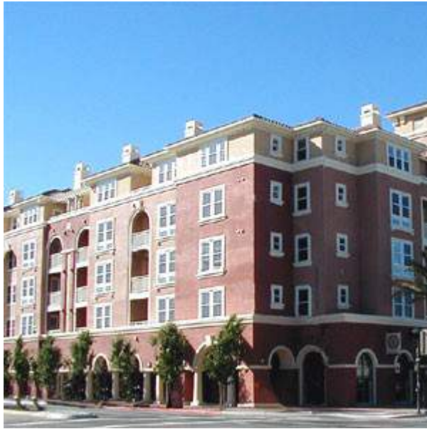
Typical Podium Building
