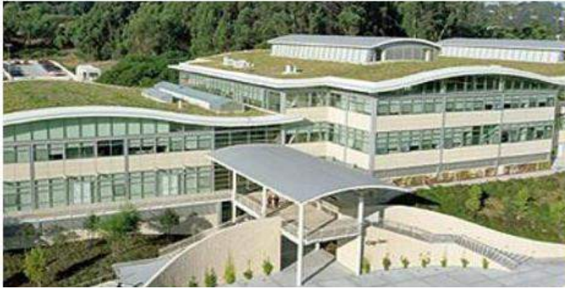
Photo 6.8-2. Extensive Green Roof at Gap Corporate Headquarters, San Bruno
