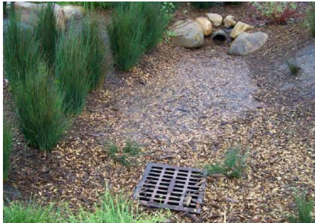
Photo 5-1. Bioretention area, Emeryville (example of a combination flow- and volume-based treatment measure)
