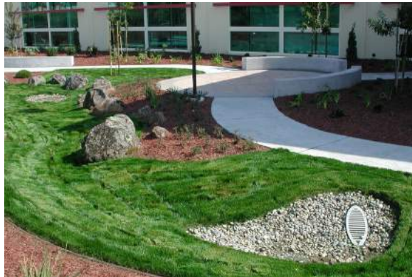
Photo 3-4. Drain rock is used to prevent erosion of this vegetated swale at Zone 7 Water Agency's office building.
