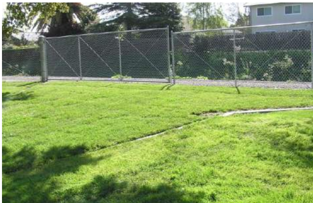
Photo 8-7. Turf block fire lane
