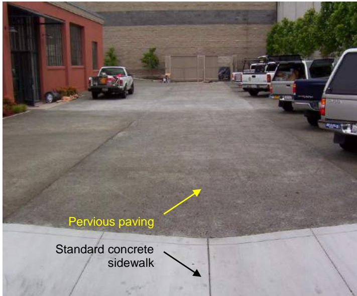
Photo 6.6-1. Parking Lot with Pervious Concrete Pavement, Emeryville
