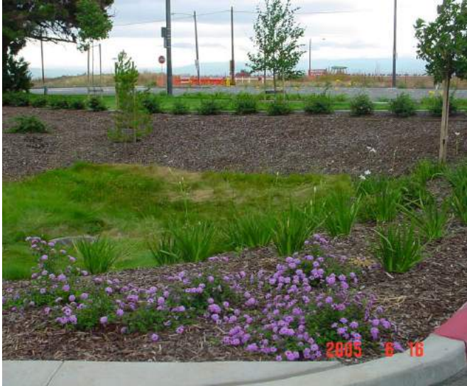
Photo 6.1-1. Bioretention area, Fremont
