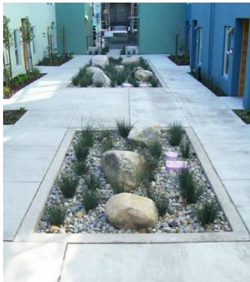
Photo 3-5. Flow-through planters are incorporated into the landscaping in a dense, urban setting in Emeryville.
