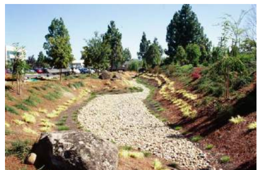
Photo 8-5. Extended Detention Basin, Palo Alto
