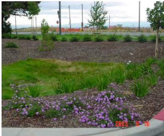
Photo 8-1. Bioretention Area in the City of Fremont
